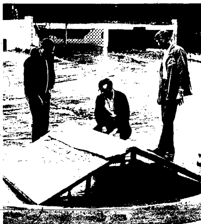
JOHN WATSON, Wayne; Dean Tietz, West Point, and Ed Harms, Wilcox, from left, observe the concrete sun drying floors for depulped coffee beans. The sun-drying floors help to reduce the moisture content of the coffee bean to 11 per cent.
